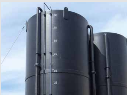
Storage tanks made of polyethylene
